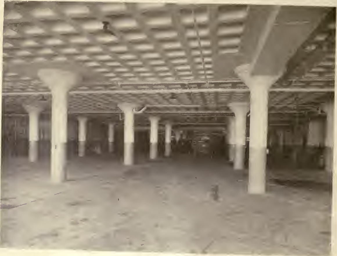
BASEMENT NOYES-BUICK BUILDING, BOSTON, MASS. ARTHUR H. BOWDITCH, ARCHITECT
